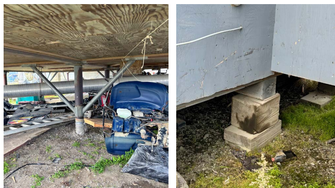
Left: Steel piles under houses in Quinhagak. Right: wood blocks under houses in Quinhagak. Photo by V. Solovyeva
